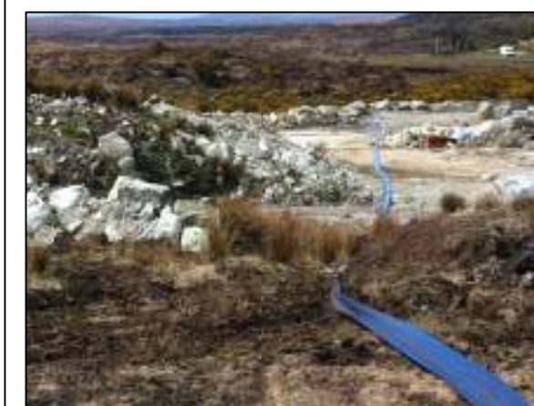
Photo 1-E Water Discharge Pipe from quarry floor.
